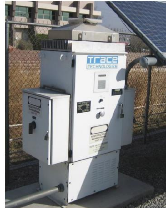
PV Inverter: DC-AC Converter
